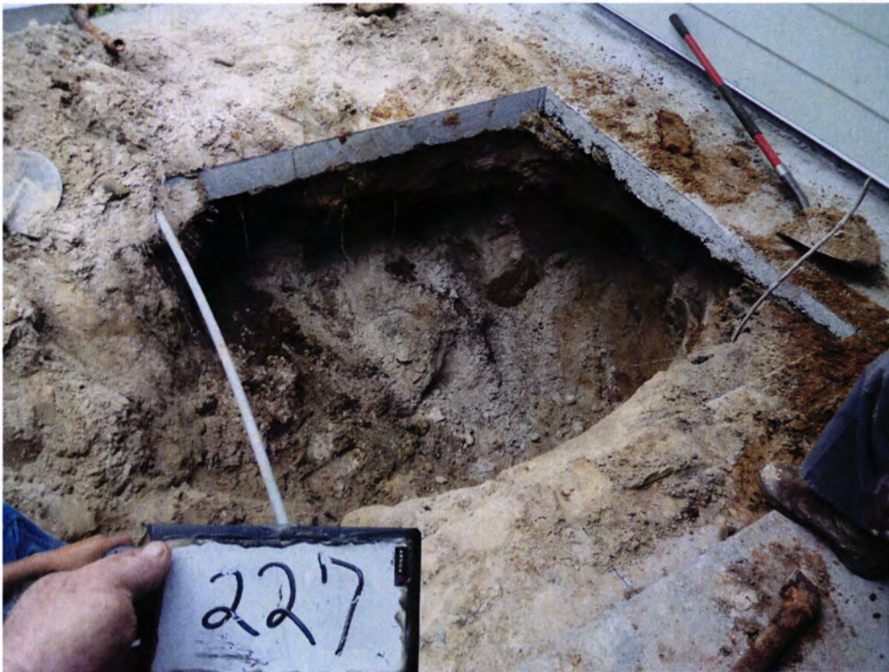
Picture 2: UST 227Cypress excavation.
